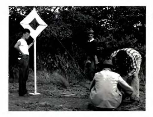
Erecting signal at Trial 193.
